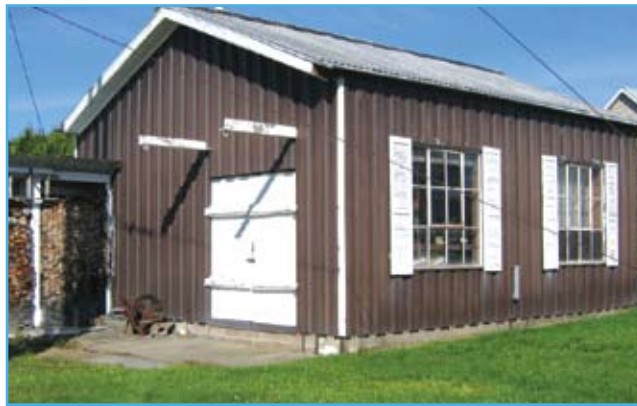
figure 1. First manufacturing building of Arcman Corporation, now used to store meters for future restoration (photo courtesy of Arcman Corporation).
